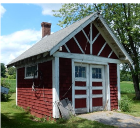
The Macedon section house as it appeared in 2015. It no longer exists.
